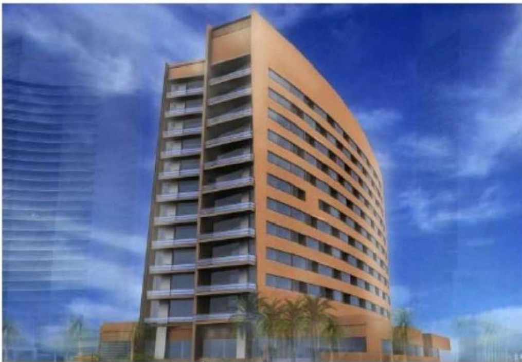
Project: 2B+GR+11 Story Residential Build Location: Plot No. 22-007 At Nad Al-Shibba, Dubai Client: Mr. Ahmed Suwadan Mohd. Al Balushi
