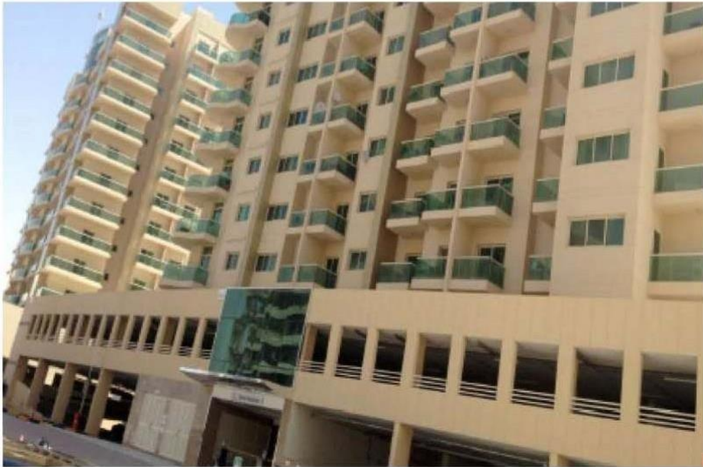
Project: B+G+P+14 Typ+Gym+Serv. Floor Resi.bldg, Location: Plot No.682-152, Sport City, Dubai
